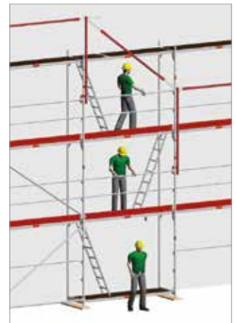
Fig. 29: Setting up the MSG front rail
