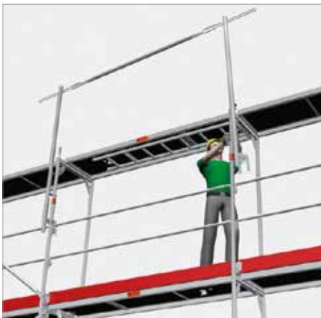
Fig. 30: Installation of the MSG in the ascent field
