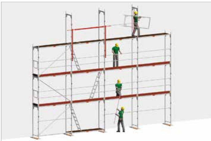
Fig. 32: Installation of a scaffold area with the aid of the PSAgA
