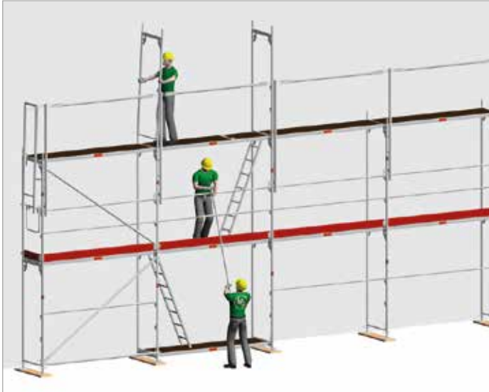
Fig. 3: Example of vertical transport of scaffold component parts manually
